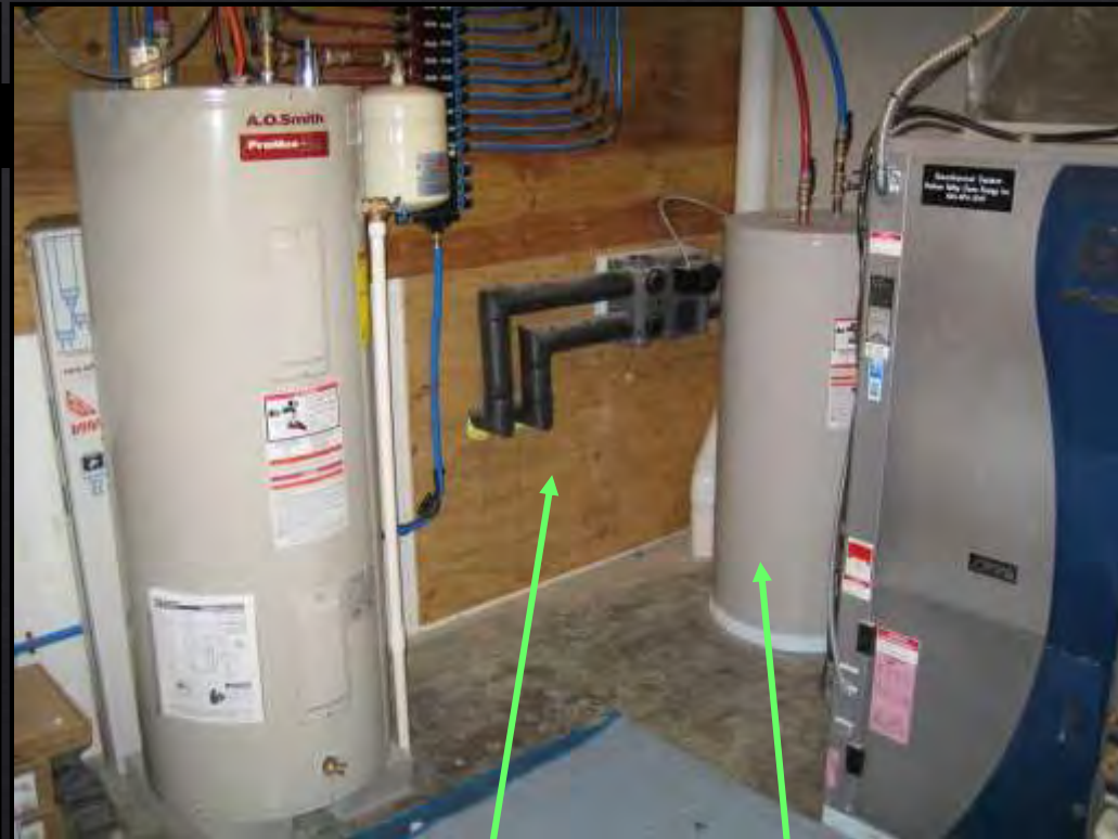
Pre-tempered water tank
