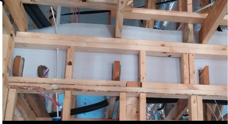
blocking between joists
