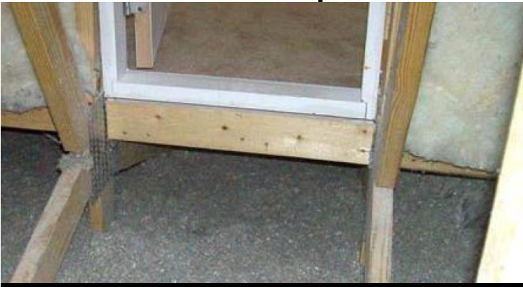
no blocking between joists
