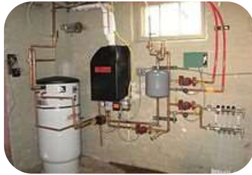
Hot Water Distribution Layout
