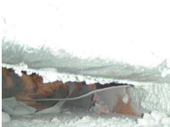
Exposed underside of duct jacket
