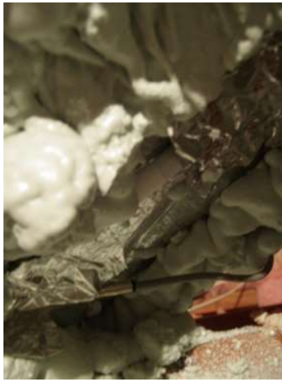
Exposed underside of duct jacket
