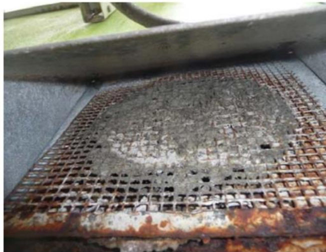
Dirty outdoor air intake.
