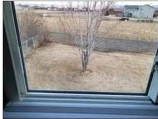
Window replaced with Thin-triple
